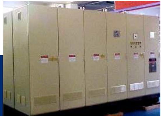
**SmartVAR™ utilizes low voltage power electronics components and capacitors as well as conventional cooling methods. This reduces complexity and initial cost while simplifying maintenance.**
